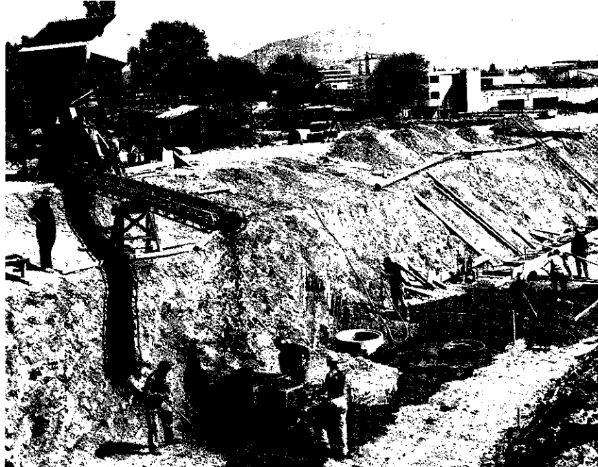
Construction of a service tunnel in progress at the beginning of June at the North East corner of the ISR site. Some of the existing CERN buildings can be seen in the background.
